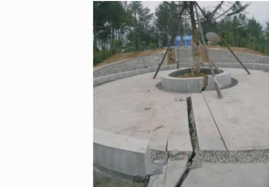
照片4 山体顶部建筑物拉裂破坏 Photo.4 Hill top buildings was tension crack
