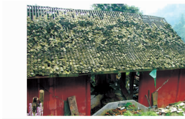
照片1 绵竹九龙乡地区寺庙屋顶破坏特征 Photo.1 Temple top building failure characteristics of Mianzhu Jiulong town area
