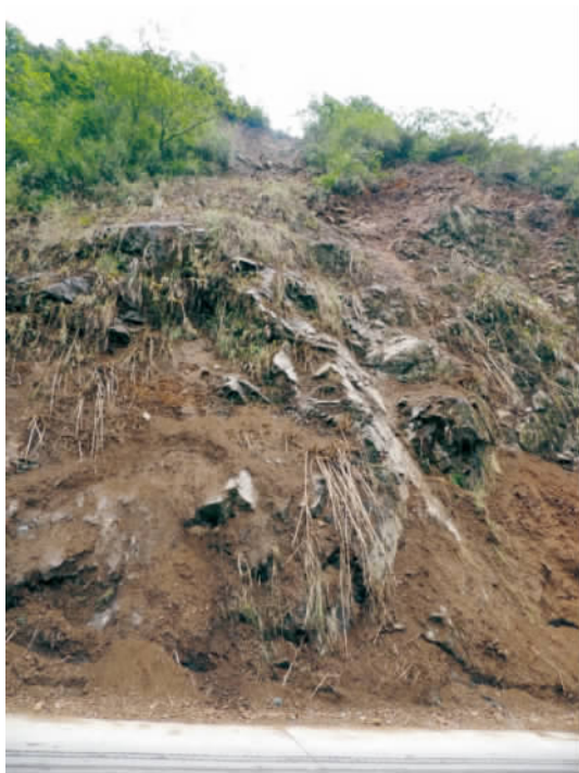
图 5 地震诱发的浅表层崩塌 Fig. 5 Collapse induced by Lushan Earthquake
