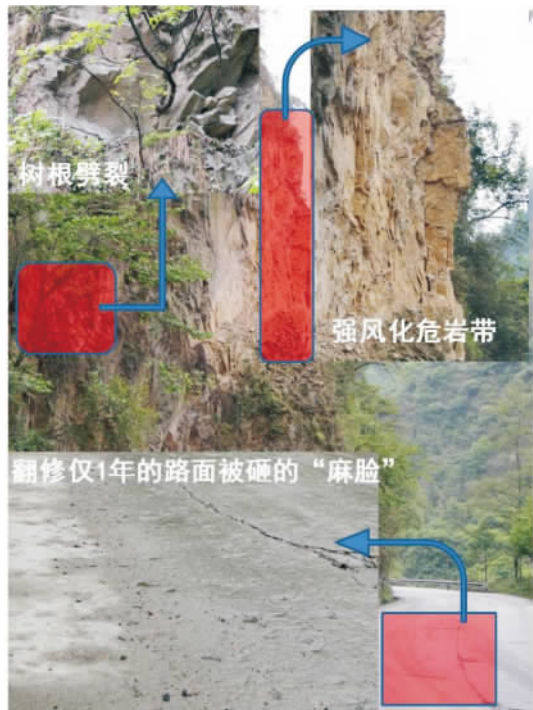
图 6 典型花岗岩崩塌特征 Fig. 6 Mantle rock and weathering residues of granite collapse
