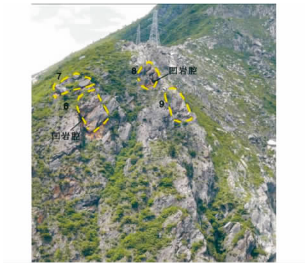
图 9 崩塌Ⅱ区不稳定危岩体及凹岩腔 Fig. 9 Dangerous rock masses and concave holes of section Ⅱ
