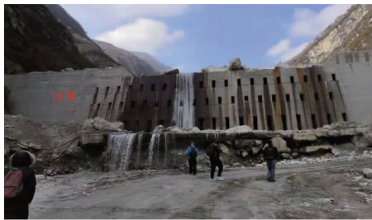
图 6 1#拦砂坝护坦冲刷侵蚀悬空(8.20 后) Fig.6 1# Sand Barrage Protector Erosion Suspension (after August 20)
